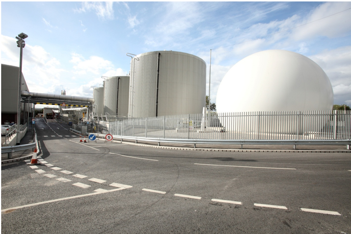
Anaerobic Digestion tanks and gas holder, Bredbury Parkway. Image courtesy of Viridor
