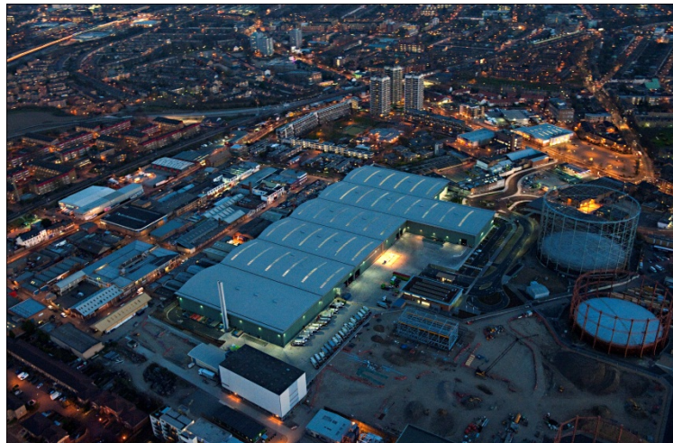
Veolia Southwark Integrated Waste Management Facility incorporating MBT and MRF. Image courtesy
